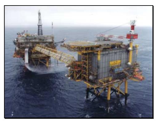
Figure 9.2 Example of a New Structure Installed Adjacent to an Existing Platform with the Potential for Gas Turbine Exhausts to Affect the Flying Environment Around New Helideck
